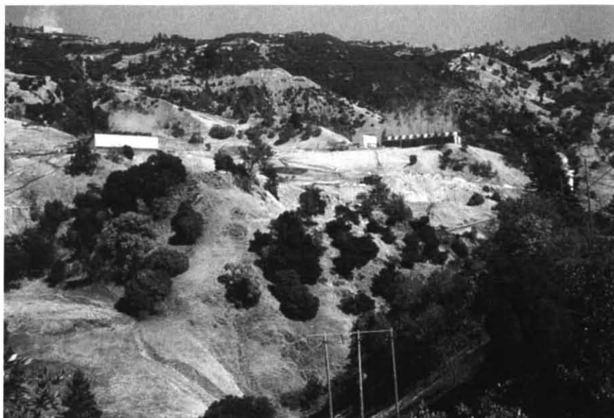
Figure 2 Three of the approximately 20 power units of The Geysers, California, USA, where electrical power is generated from a dry-steam resource.
